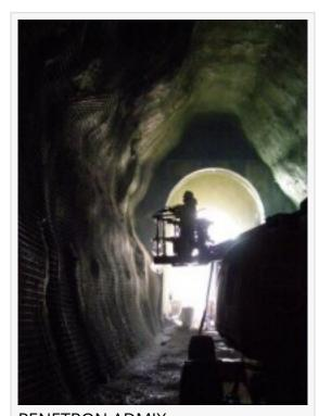
PENETRON ADMIX was incorporated into the ready-mixed shotcrete material at the time of batching and was placed pneumatically to waterproof and structurally reinforce the tunnel for years to come.
