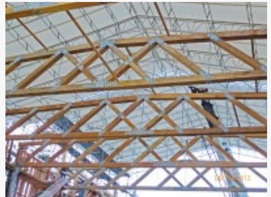
Giant structural timber trusses in San Francisco's Pier 29 boat shed were designed, built, and delivered by American Pole and Timber in Houston, TX.
