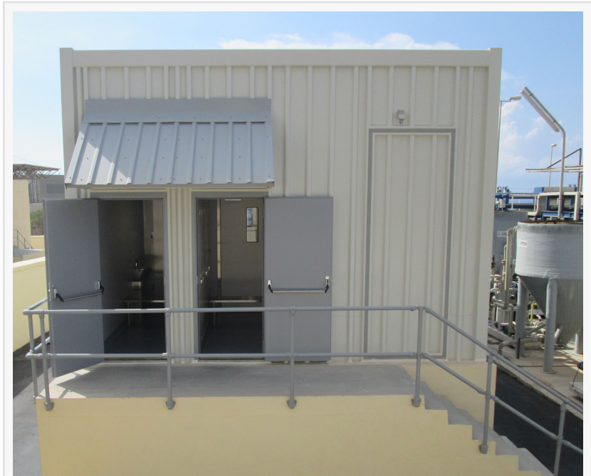
The modular laboratory has been built as a single structure that comprises nine rooms grouped in four areas
