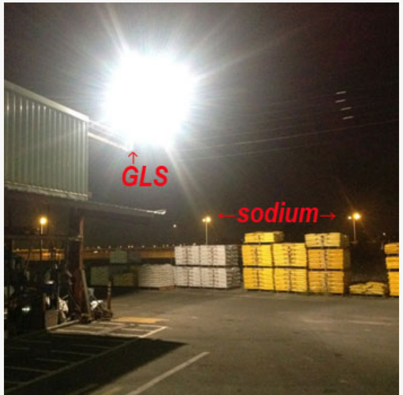
Construction site with GLS compared to regular sodium (HPS)
