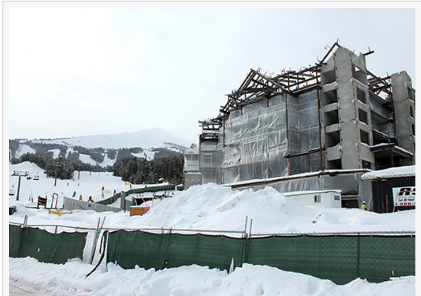
The Grand Colorado on Peak 8 under construction.
