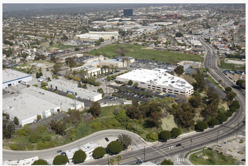
Grifols Los Angeles Manufacturing Facilities
