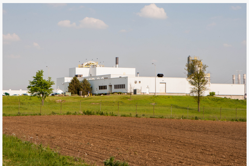
The Nutrinsic Protein Production Facility co-located at Miller Coors Water Reclamation site
