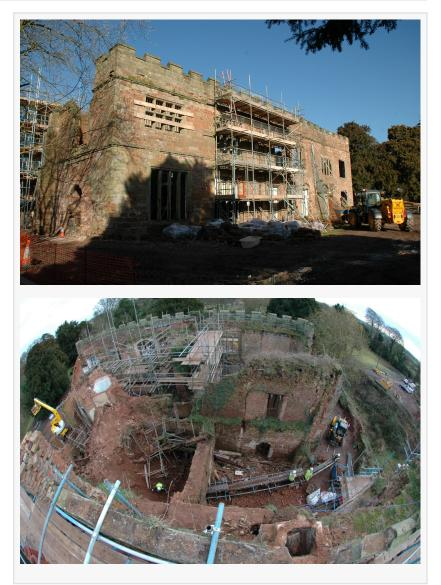
pumped out. Cores removed during this process were retained and reused where the anchors were installed, leaving an almost invisible repair. The work has ensured the survival of the original walls, allowing the award-winning holiday home to be built within the shell of the ancient castle.
