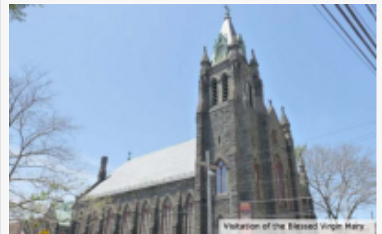
Bronx-based Start Elevator restored a 19th century church's elevator for free, after Hurricane Sandy left it out of service for more than two years.
