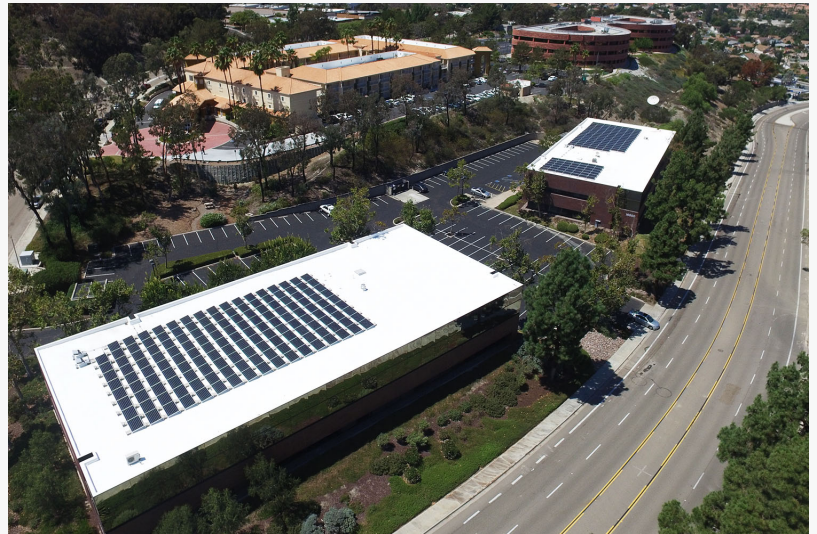
Bernardo Views Ballasted Solar System
