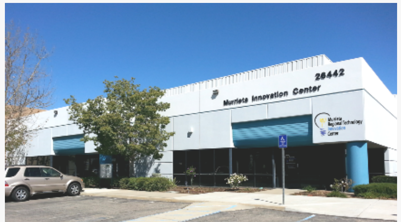
Murrieta Innovation Center
