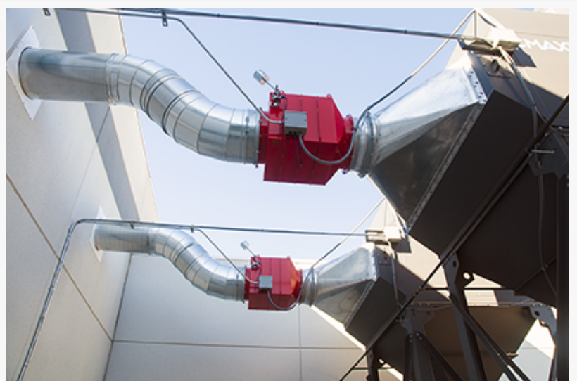
These Explosion Isolation Valves give added protection to our customer's facility
