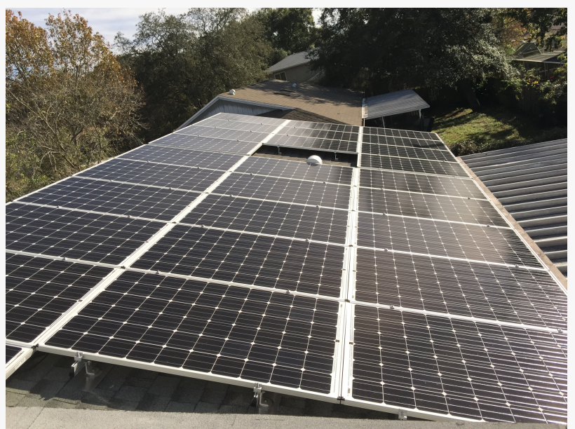
Tampa Solar-Panel Installations
