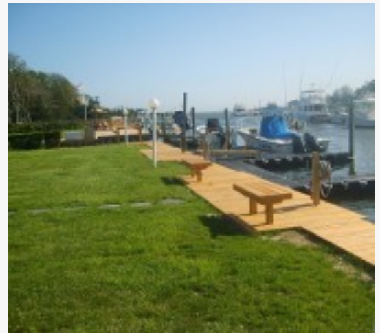
Marina in Hampton Bays, Boat Slip Hamptons, NY
