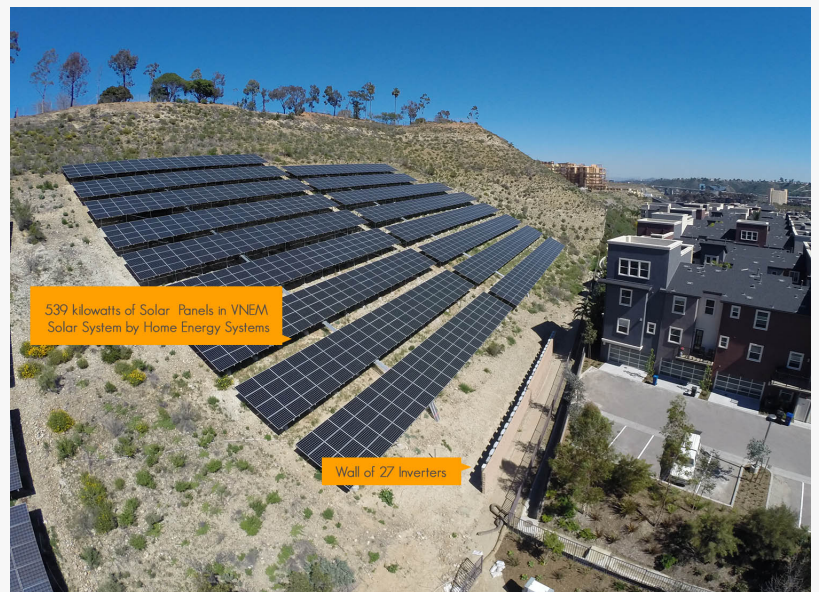
1,648 panel, 536 kW of VNEM Solar Systems by H.E.S. Solar
