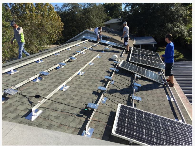
MC2 Solar's Residential Solar Panel Installations
