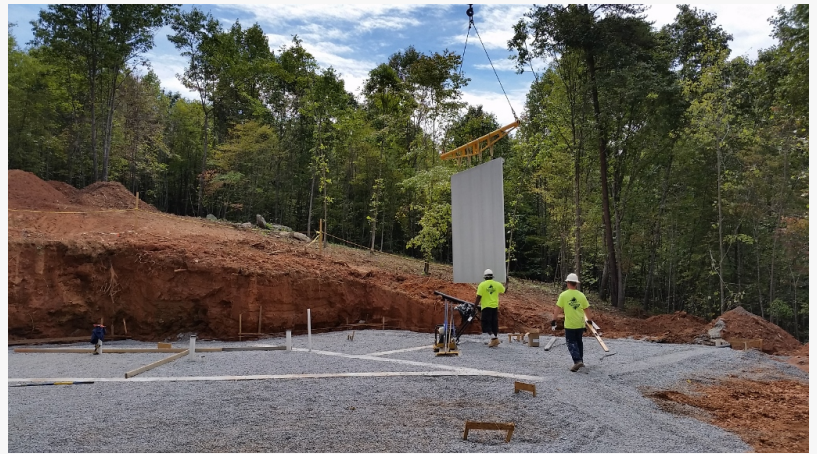
S. D. Jessup Construction team installing precast Superior Walls foundation panel.
