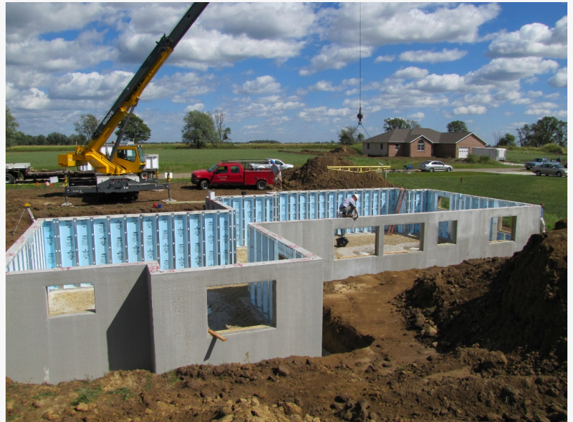
Installation of a Superior Walls precast concrete foundation system.
