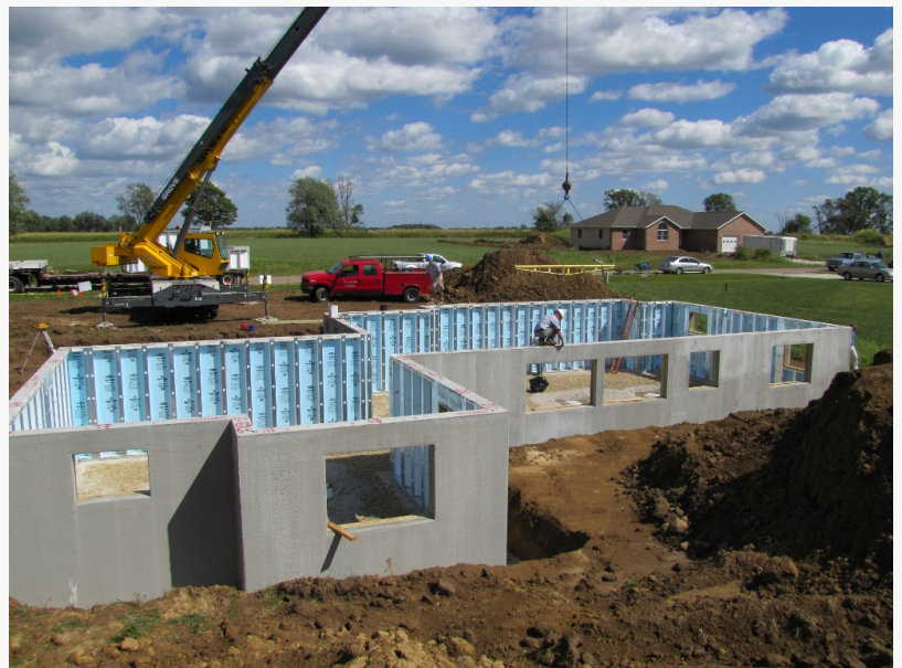
Installation of a precast concrete wall foundation from Superior Walls.
