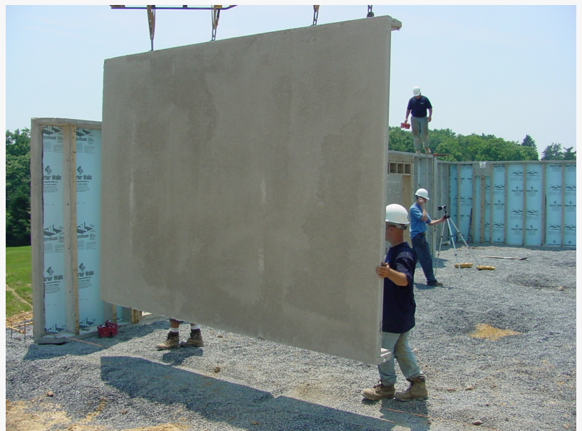
Superior Walls foundations being placed on jobsite.
