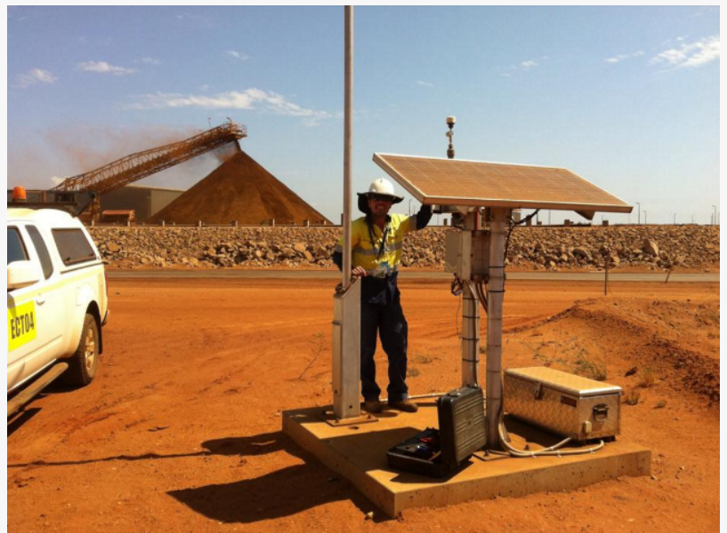
Solar powered particulate monitor in Port Hedland, WA. Ecotech Technical Support Specialist, Nuno Rodrigues, performing site maintenance.
