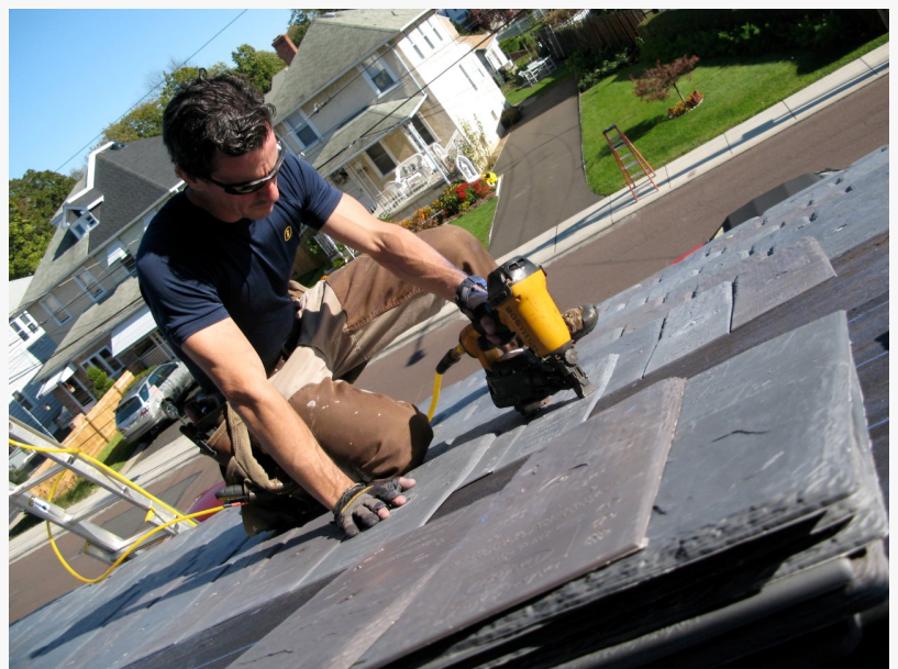
Installation of DaVinci Roofscapes synthetic roofing tiles.
