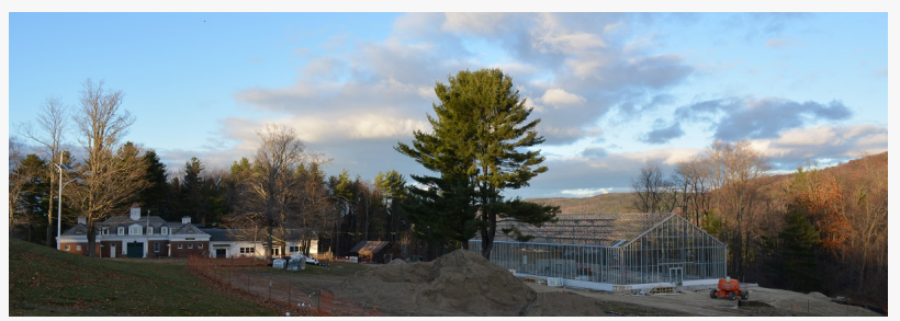
Eco-water reclamation housed in a giant green house by Tallyho For school visits and various eco-tour
