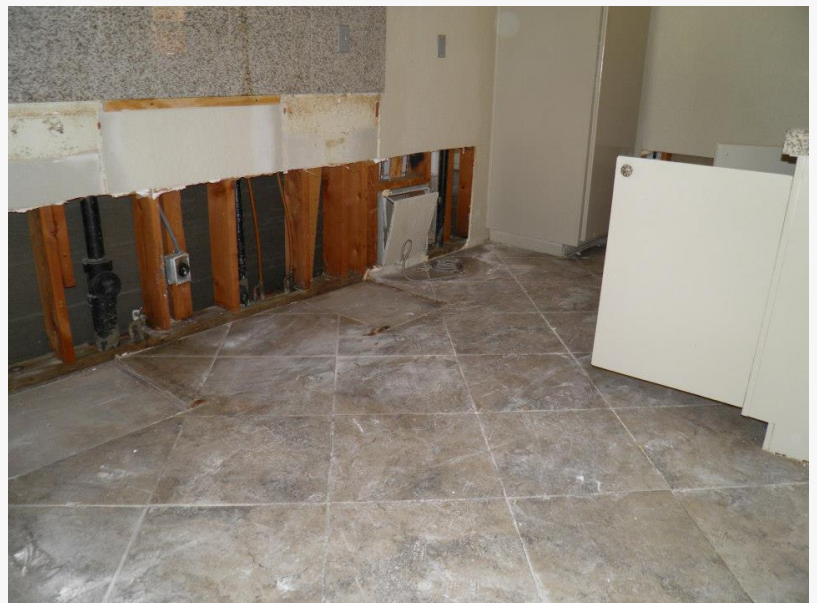
This Is What Water Damage Does
