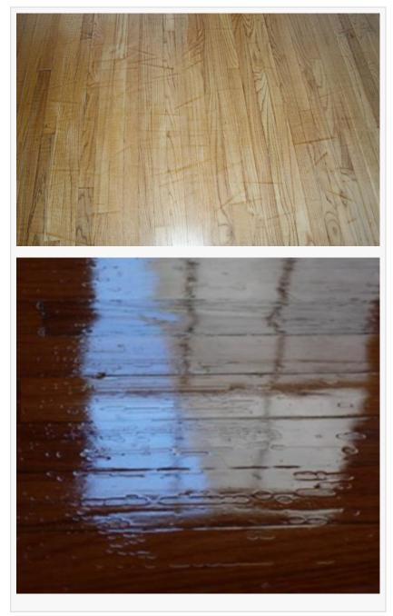
The wrong type of adhesive, trowel and or spread rate of the boards when they were installed or it could be poor manufacturing of the wood boards themselves. For factory-finished flooring, simply correct the problem by replacing the boards that were not good. For un-finished flooring, correct the problem and then re-sand the floor to smooth the levels out properly, if necessary.
