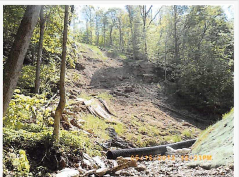
Dominion pipeline in West Virginia
