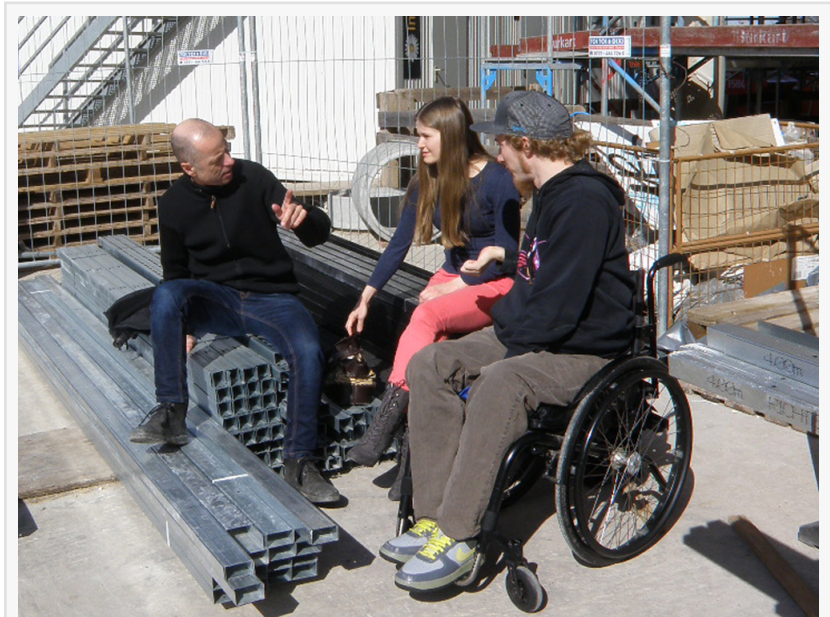
Wolfgang Frey in conversation with future residents at the construction site for Heidelberg Village
