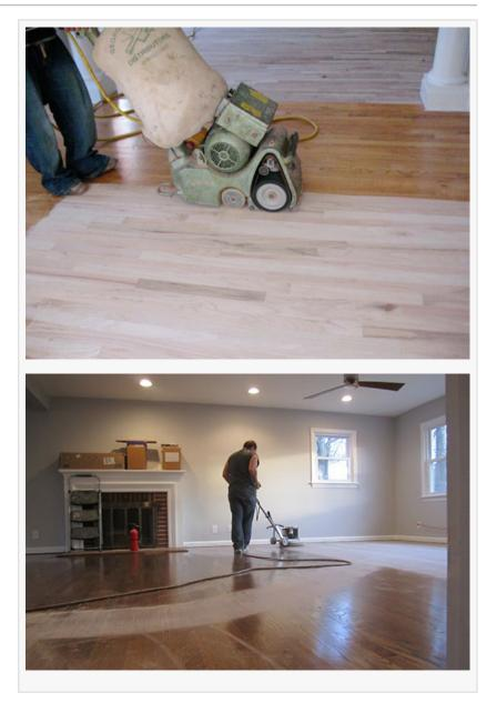
Yearly wear is a problem. It is typically caused by improper floor maintenance that fails to remove grit from the floor, or the introduction of water or strong cleaners. Pet nails and unprotected furniture legs also contribute to the problem. Proper maintenance requires regular dust-mopping with an approved wood floor cleaner. If re-coating is necessary then you might want to consult a professional floor company.
