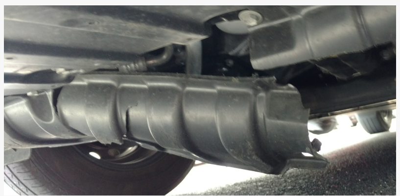
Under car damage could result in driving hazard and liability
