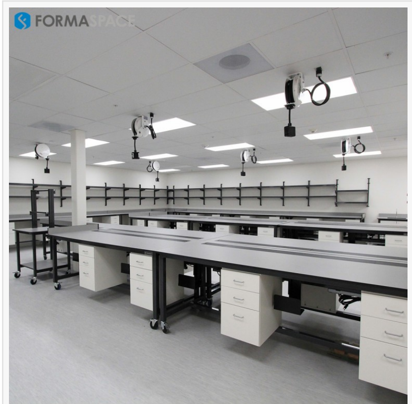
Ariosa Modular Wet Lab Installation
