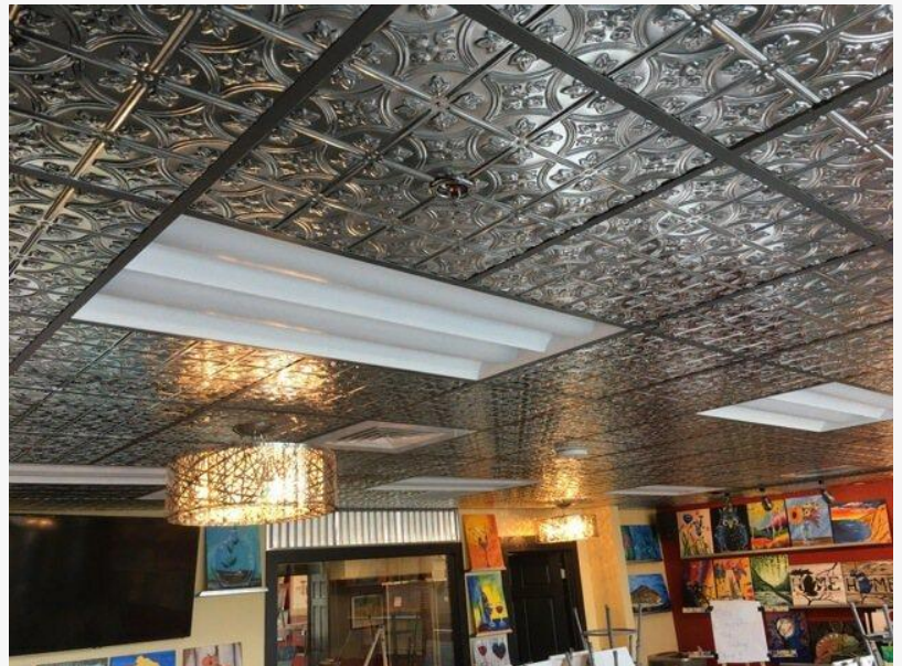
Suspended ceiling in a Victorian design
