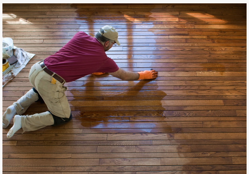
Refinishing a hard wood floor
