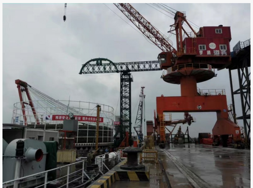
Hengtong(Changshu) Harbor Dock
