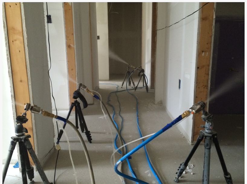
Multiple spray nozzles can be used to quickly and effectively seal the building envelope of entire structures.
