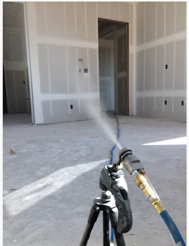
AeroBarrier is applied as an aerosol mist of sealant that seeks out and fills leaks throughout the entire building envelope
