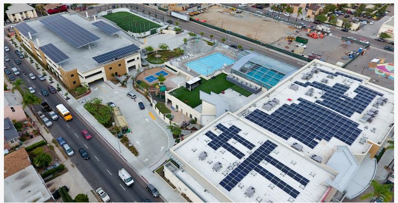
Home Energy Systems installed a large commercial solar panel system on the YMCA in San Diego. Adding to their success this past year.
