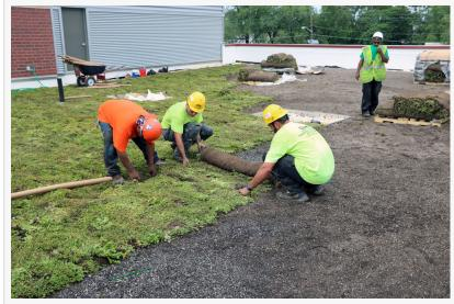
In the construction of this new facility, the green roof presented a very economical and environmentally friendly stormwater solution.
