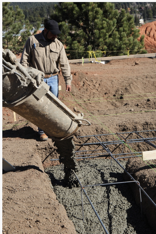
First concrete pour (Photo by CR Chambers Photography)
