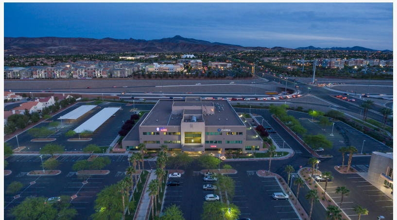
Medical Plaza Parkway Exterior
