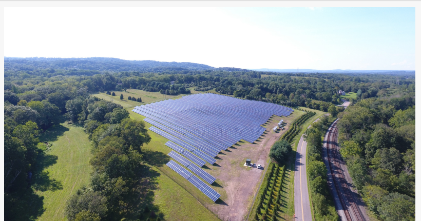
Fischer Solar Farm
