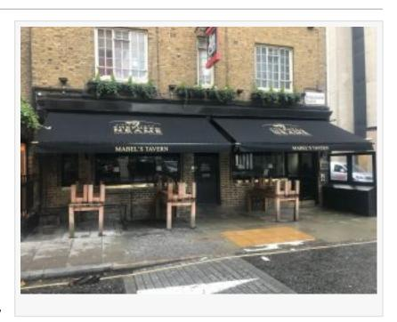
wood and slowly eat into it. Radiant Blinds still use hardwood cheeks and a timber front lath and tacker. The arms are designed to suit the exact requirements of the building and are bent by hand as they were during the time of Queen Victoria. The Victorian awning is operated with a traditional pull down pole.
