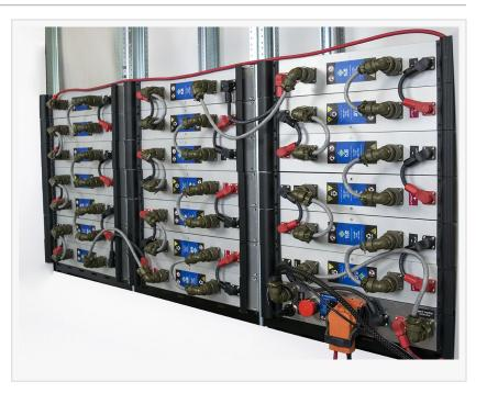
powerful battery management system designed and developed by K2. The second module is the battery module that allows for customizable amounts of power storage. Each battery module is protected with internal fuses and has cell monitoring boards that have voltage and temperature sensing as well as balancing.
