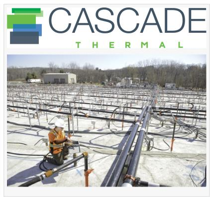
The technology offering and proven performance record distinguishes Cascade Thermal among in situ thermal remediation providers. No other competitor has the history of successful implementation of all three of the most commonly used forms of subsurface heating technologies: Thermal Conduction Heating (TCH), Electrical Resistance Heating (ERH), and Steam Enhanced Extraction (SEE).
