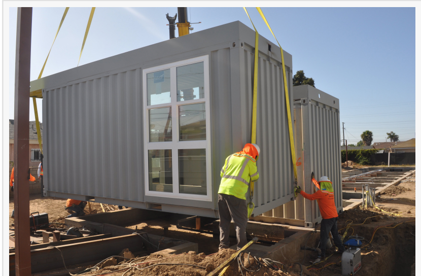
The first story of FlyawayHomes installation.
