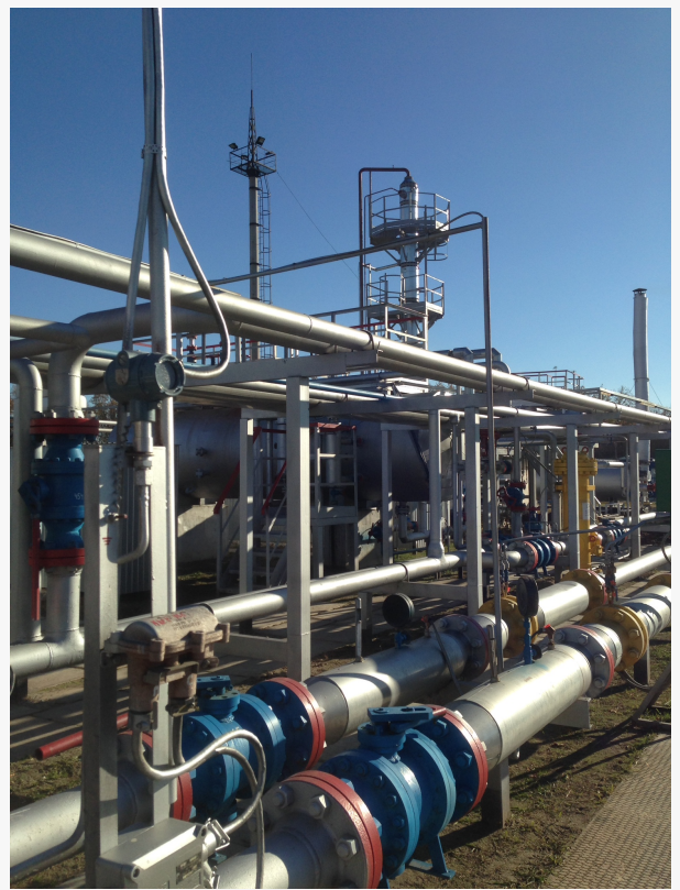
Burisma Group Announces Construction of a Condensate Stabilization Unit for an in-depth Propane-Butane Mixture Extraction on Vodyanivska Area
