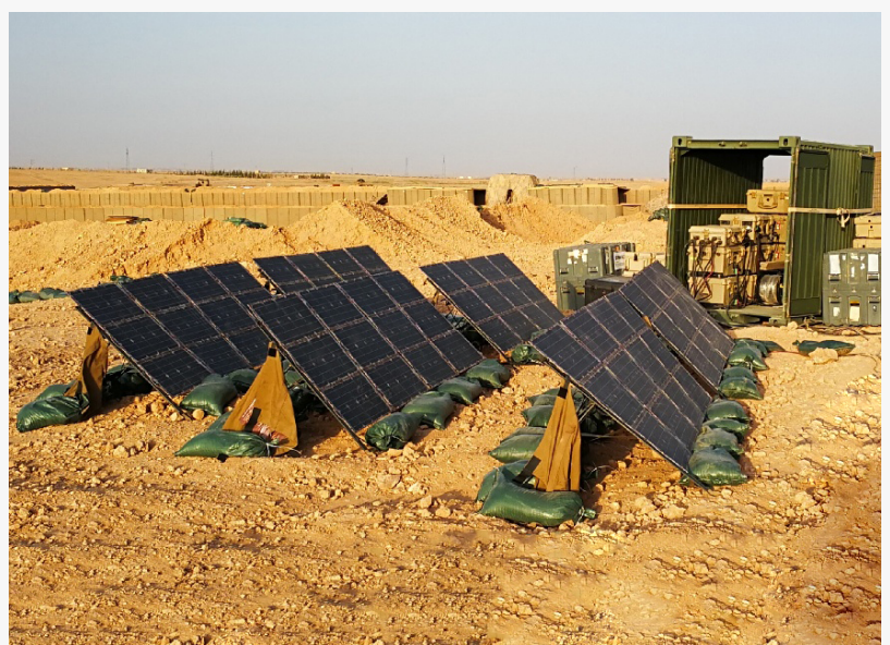
An Alternative Energy System (AES) is shown deployed at a combat outpost in the Middle East.
