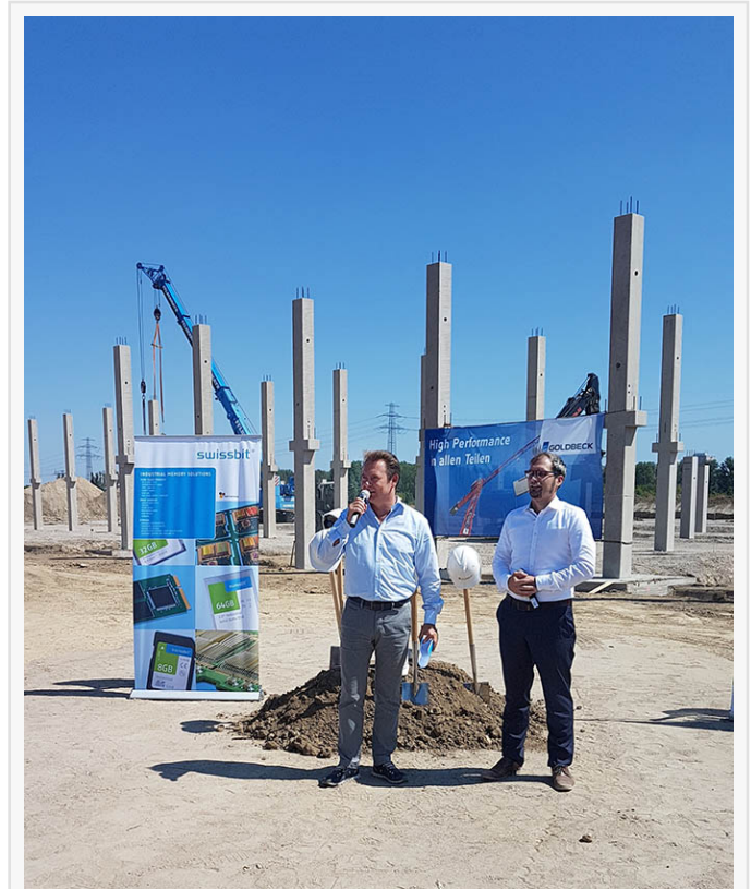
Silvio Muschter (CEO, Swissbt AG) and Johannes Martin, District Councilor & Head of Department for Economics, Roads and Green Spaces, ceremoniously initiate the construction of the new Swissbit manufacturing plant.
