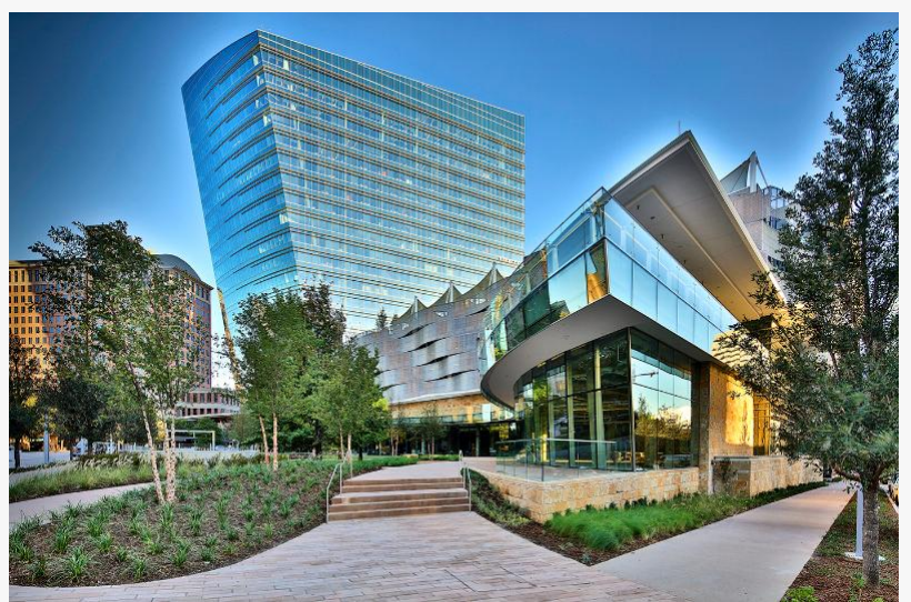
The Pelli Clarke Pelli Architects design McKinney & Olive provides a welcoming street-level view in pedestrian-friendly Uptown Dallas.
