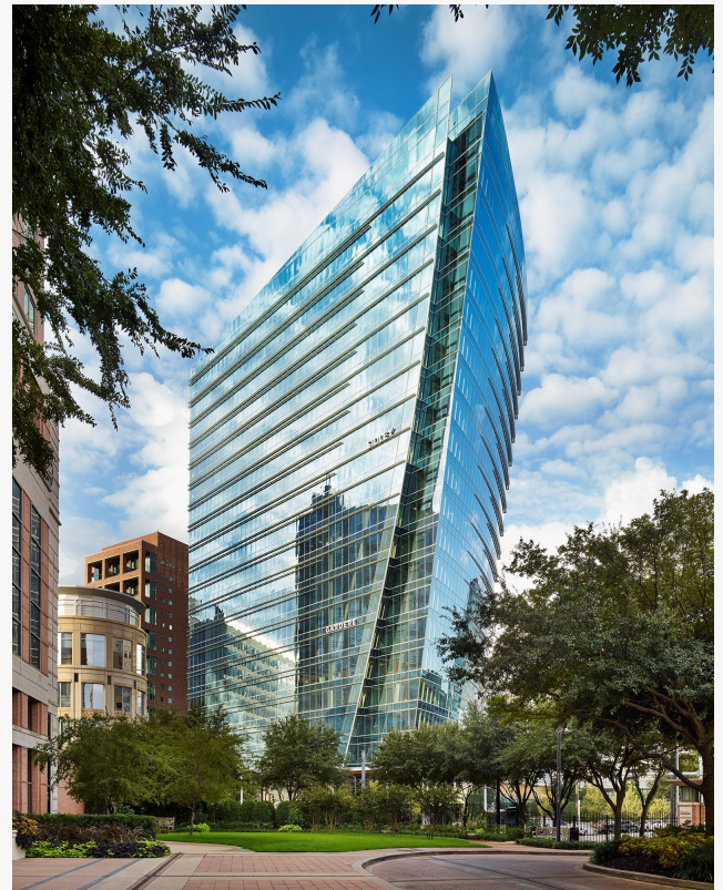
The Pelli Clarke Pelli Architects "sexy design" McKinney & Olive is now 100 percent leased.
