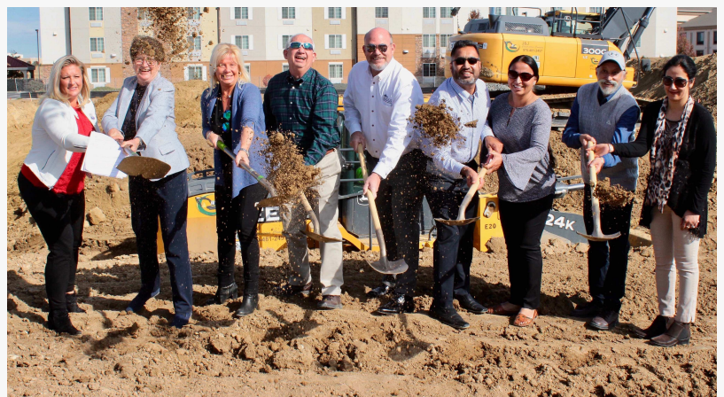
Loveland, Microtel, Construction and Owners participate in groundbreaking. Photo by Melissa Stewart (perini & associates)
