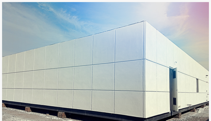
Modular Solutions factory
