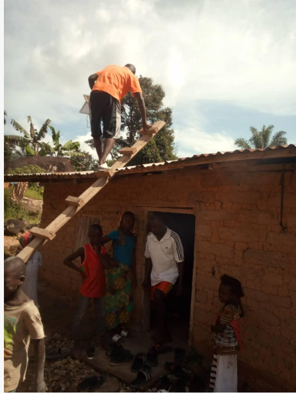
Ignite Power engineer installation a Solar System on a home in Karyadu
