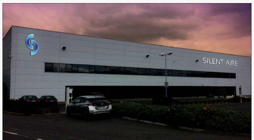
Silent-Aire EMEA expansion at 56 Park West Road Park West Industrial Park Dublin 12
