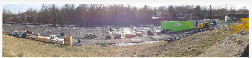
Installation of thermal remediation system at inactive hazardous waste disposal site
